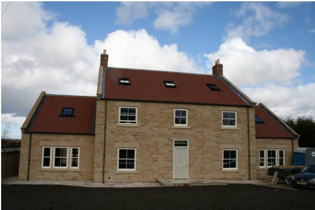
Front South Facing Elevation of St Hilda's House.
